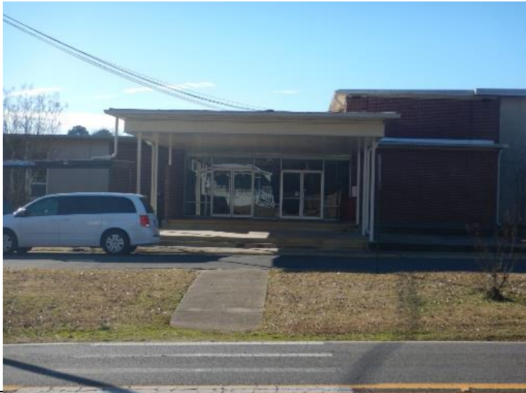
Property 26a, North Side (Entrance)
