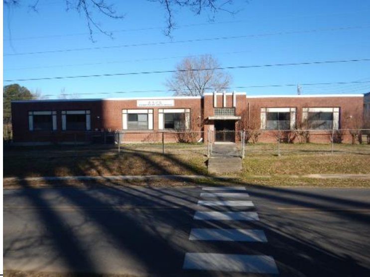
Property 26f, South Side
