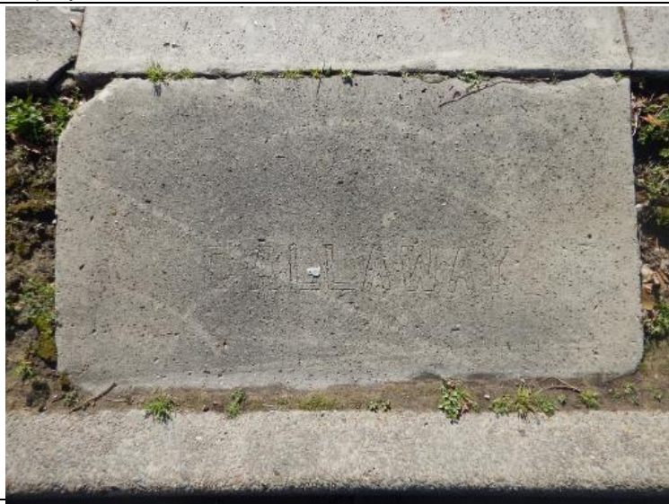
Property 44/CL0068, Stepping Stone Near Curb
