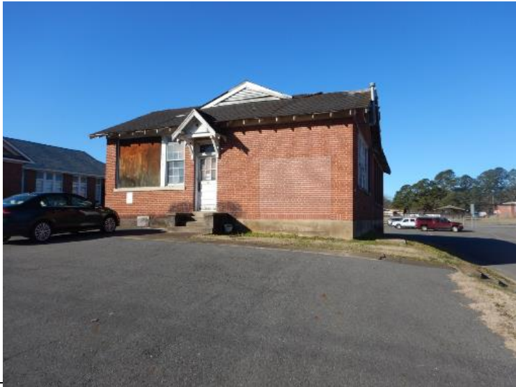
Property 26d\CL0947, East Side
