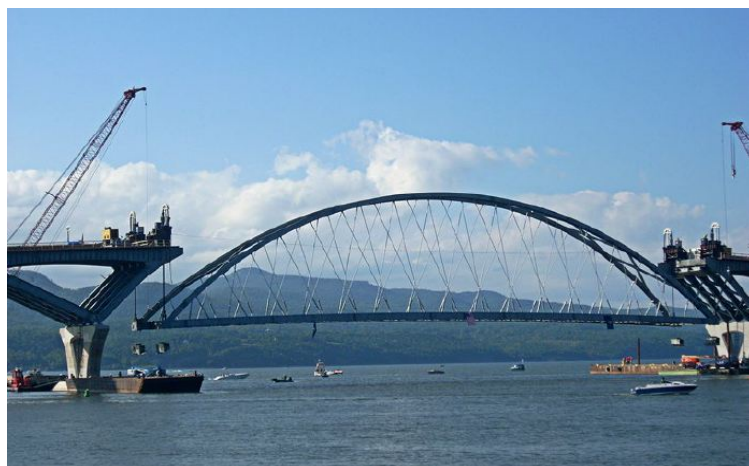
The new Lake Champlain Bridge, which features a 402-foot arch floated into place over the course of 18 hours, opened to traffic in November 2011. (Courtesy of NYSDOT)
