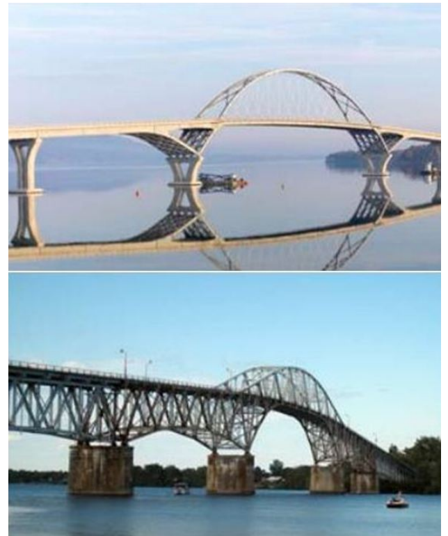
In response to public input, the lead agencies selected the design option (top) that recalls the original 1929 bridge (bottom). (Courtesy of HNTB)
