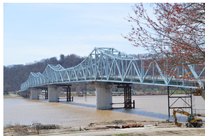
The bridge after the slide was completed. (Courtesy of FHWA Indiana Division Office)
