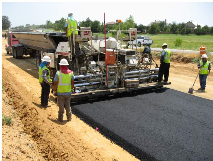
Warm-mix asphalt pavement construction is an example of a technology that can increase the sustainability of pavement systems. (Courtesy of FHWA)
