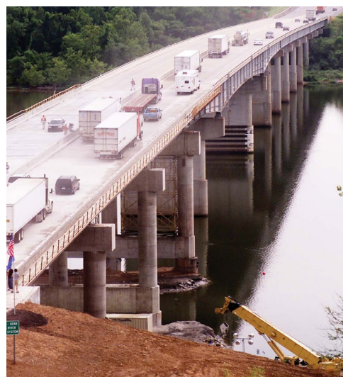
Figure 9 New I-40 Bridge
