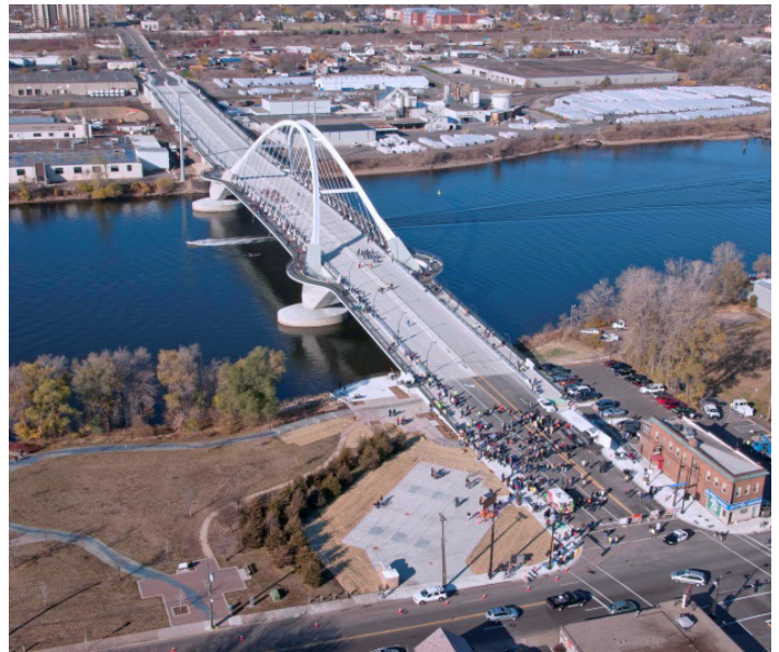
The new Lowry Avenue Bridge in Minneapolis, Minnesota—another 2013 EEA winner—uses innovative water quality practices to protect the Mississippi River from harmful pollutants and runoff. (Courtesy of FHWA)
