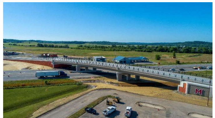
Figure 3. Grand Valley Boulevard Bridge in Martinsville, Indiana. Source: INDOT.
