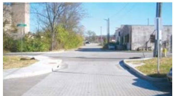
Johnson Street in Chattanooga before (top) and after (bottom) the redesign addressing flooding risks while providing a bicycle- and pedestrian-friendly green street (image courtesy of FHWA).
