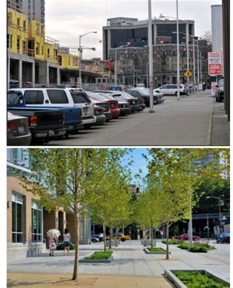
Taylor Avenue North in Seattle before (top) and after (bottom) the redesign project providing both space for bicyclists and pedestrians and stormwater management (image courtesy of FHWA).
