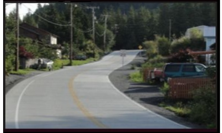
The top photo shows the roadway prior to the start of the Shtax'Heen Roadway Improvement Project. The bottom photo shows the completed roadway. (Courtesy of the WCA)
