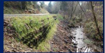
Figure 1: Mechanically stabilized earth. Photo credit: Oregon DOT
