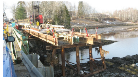
Typical trestle/temporary bridge construction. Image courtesy of MaineDOT.
