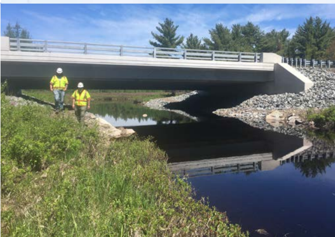
Before (top) and after (bottom) Pembroke Stream Bridge replacement (Courtesy of MaineDOT)
