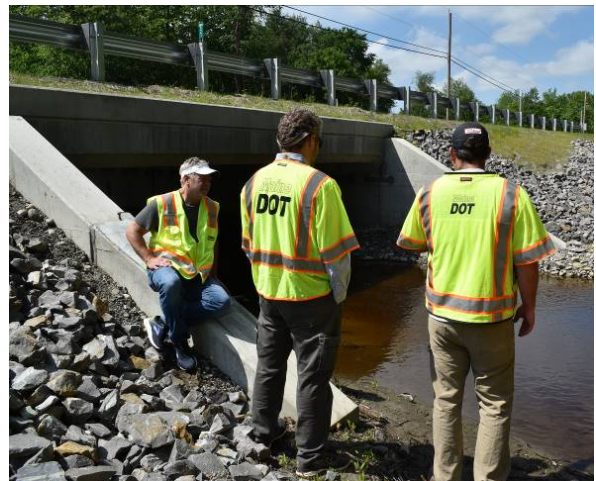
Staff from MaineDOT, USFWS and FHWA inspect a completed culvert replacement in Sidney, ME (FHWA/Volpe)
