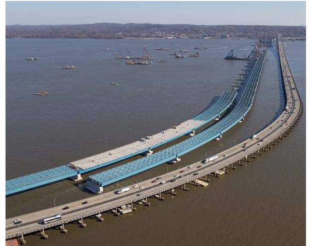
Tappan Zee Bridge under construction (courtesy of New York State Thruway)
