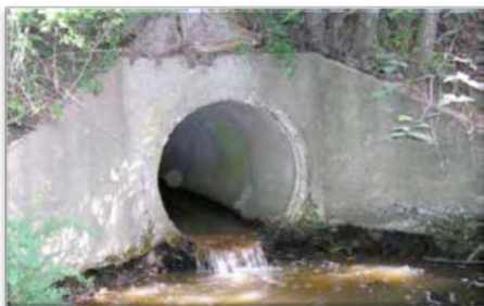
Undersized crossings restrict natural stream flow and can cause problems during floods. (Courtesy of TNC)
