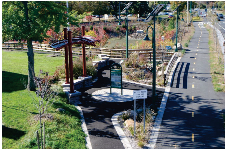
A focus on sustainability and collaborating with transportation users led NYSDOT to add new transportation features during a reconstruction of Route 347, including a greenway stop, rain garden, information kiosk, and recharge basin. (Courtesy of NYSDOT)
